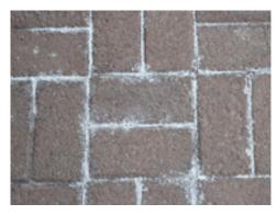
Salts and minerals leaching out of concrete basements or walls form a white, powdery crystals called efflorescence. Sometimes it may be difficult to visually distinguish between efflorescence and mold. However, since efflorescence is caused by water problem there are chances of mold growth too.
