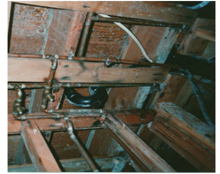
Figure 4. Mouldy ceiling wood. Use tape lift or contact plates (or swabs) to sample visible mould like this.
